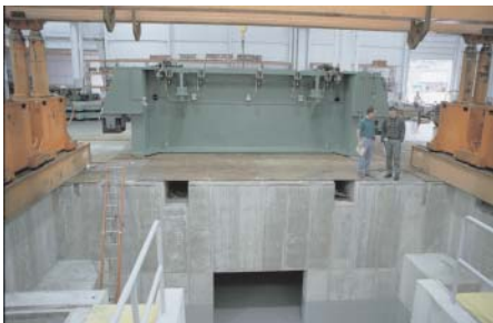
The press bed is ready to be installed into the pit.
